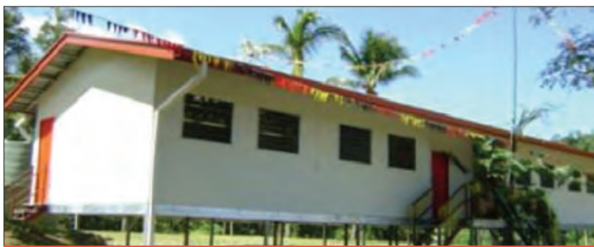
One of the double classrooms the Digicel Foundation is building for schools
