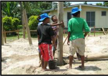
Female carpentry students putting up posts for a new building
